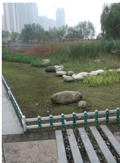
A rain garden taking footpath runoff
