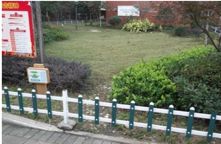
An example of a swale (swales are shallow, broad and vegetated channels designed to store and/or convey runoff and remove pollutants) near residential housing in Wuhan
